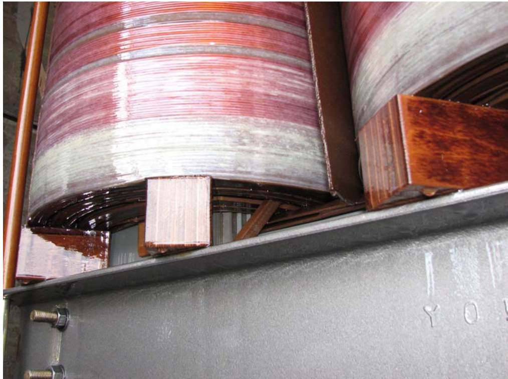
Fig. 7 Exemplary photograph (phase C) of small distance sticks of stray channel between HV- and LV-winding
